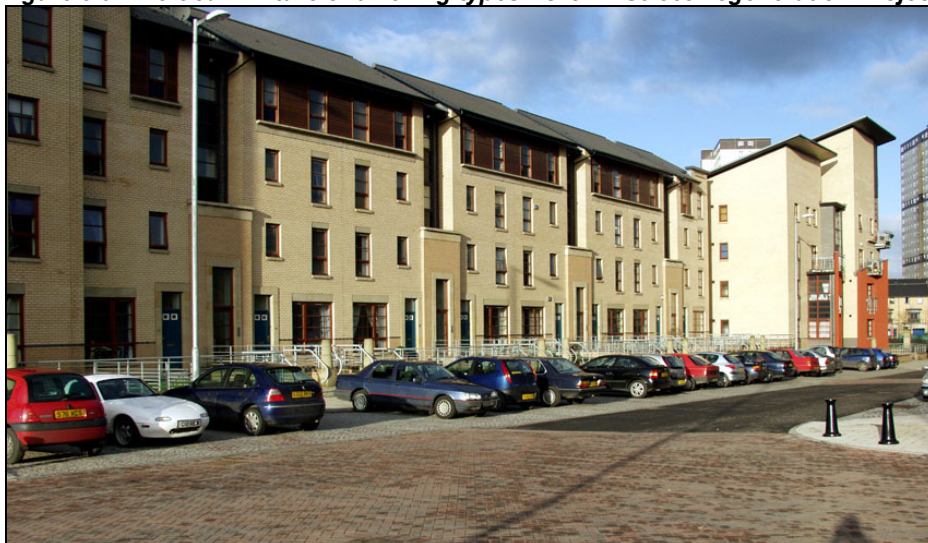
Figure 3.04 Vertical mixture of dwelling types - Crown Street Regeneration Project, Glasgow
