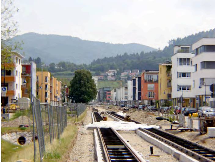
Figure 5.11 Tram route extension under construction at Vaubanallee (2004)
